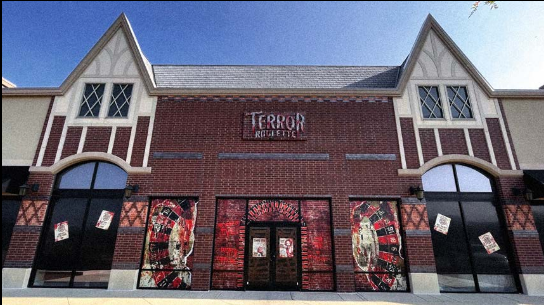
FABRICATED WINDOW VINYL & SIGNAGE
